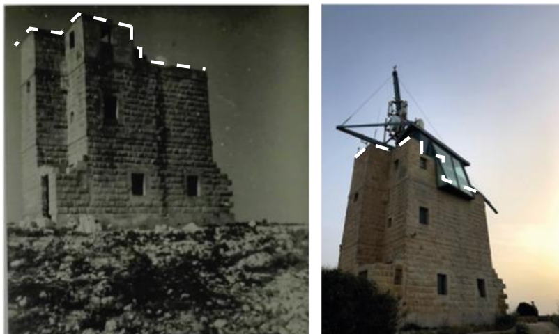
Figure 62: The line of destruction is the original outline in Ta' Kenuna Tower. Image source (left): Nadur Local Council; (right) photo by author, taken 14 June 2019
